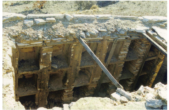
Fig. 14 "Melissokipi". The "cupboards" clearly seen as the roof has collapsed (photo: G. Speis).
